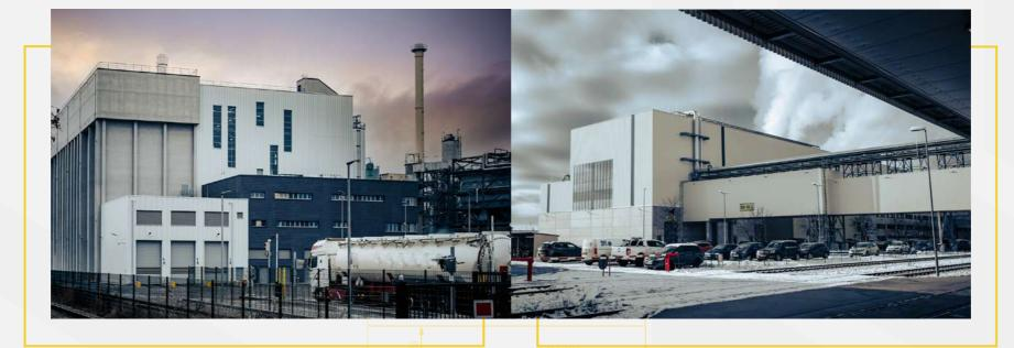
The sewage sludge utilization plant in Bitterfeld plays a central role in Germany's phosphorus recovery strategy, disposing of approx. 260,000 tonnes of sewage sludge annually. The process of thermal utilization allows the recovery of phosphorus from the ash, which is an important step in closing the phosphorus cycle. The plant is self-sufficient in terms of energy and even produces renewable electricity.
